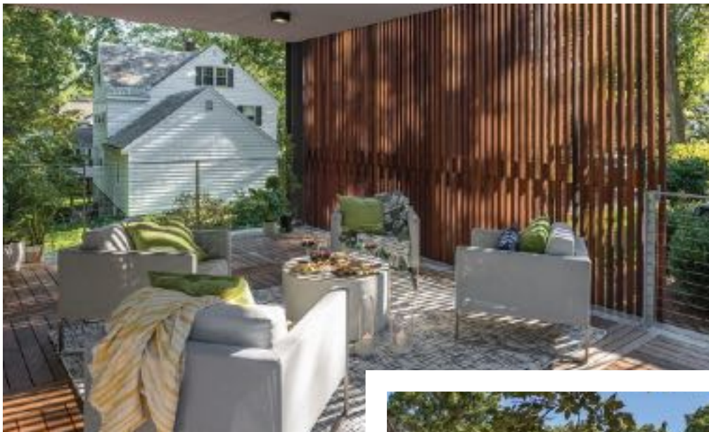
From top: The middle floor, set a few steps above the backyard, is an open-air veranda that gets its privacy from the street by a three-level mahogany screen; the lowest level of the structure, set into the sloping site, contains a 670-square-foot garage workshop, where the homeowner repairs antique Vespa scooters.
