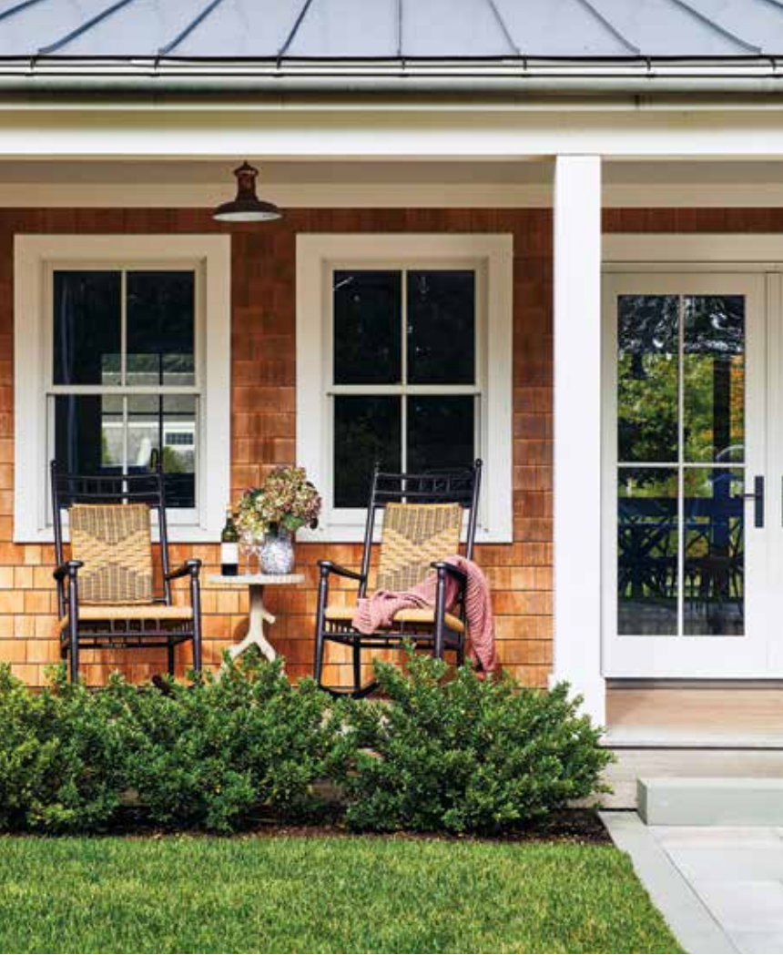
ABOVE: The home's standing-seam aluminum roof matches the roof on the nearby barn. "It's a nod to a simple agricultural metal roof," says architectural designer Tom Carberry. BELOW: In the living room, wainscoting, Designtex grasscloth wallcovering, and a trunk-turned-coffee-table make the home feel older than its two years. FACING PAGE: The fireplace mantel was crafted from the same reclaimed yellow pine as the floors. "The mantel was something the homeowner was passionate about," says designer Jesse Carrier.
